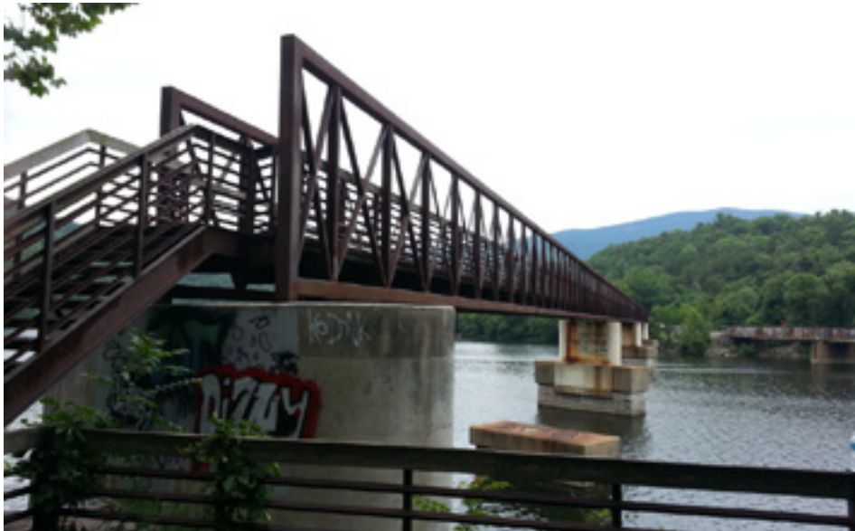
Footbridge over the James River
